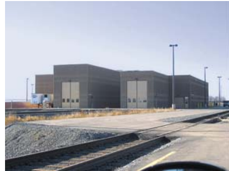
The MTU Onsite Energy standby power system provides support for the vehicle maintenance facility's electric loads, including HVAC systems and large-scale industrial equipment for maintenance and repairs.
