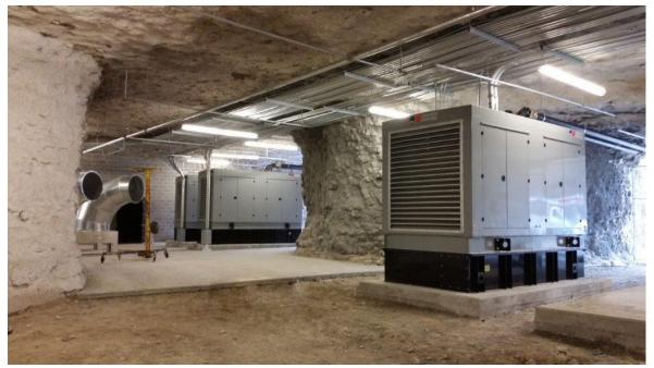
Cavern Technologies recently installed three new MTU Onsite Energy generator sets producing 500 kWe for their newly-expanded datacenter near Kansas City.
